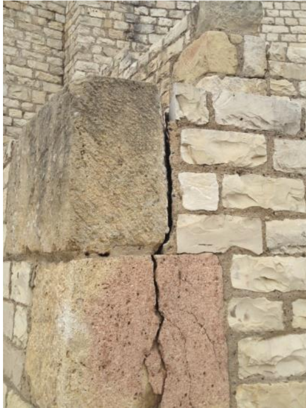
Figure 10. Detachment, the Archaeological Ensemble of Tárraco (Spain)
