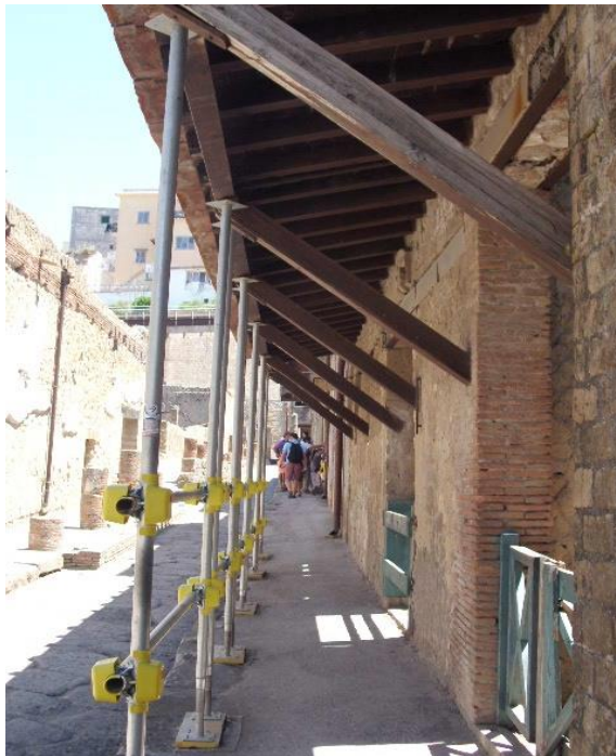
Figure 3. Static weakness, Herculaneum (Italy) archaeological site
